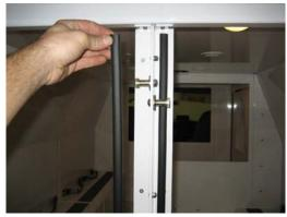
Cut door gasket with utility knife. Cut gasket to the length of door acceptor frame. Attach as shown above.
